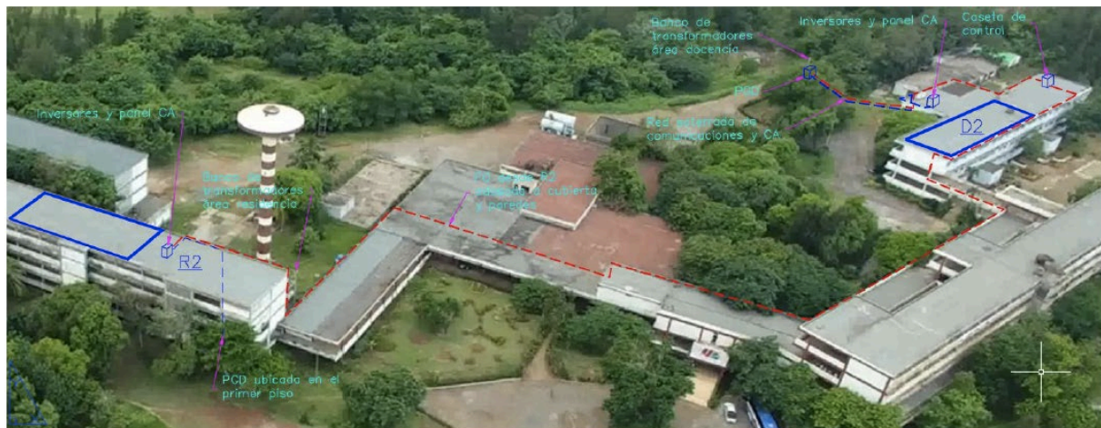
Figure 1: Aerial view of the rooftops for SDS installation
